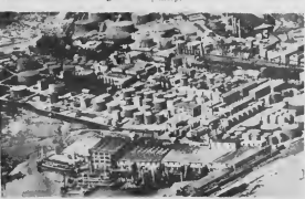
NO LONGER a part of the Standard Oil Co. (N.J.) is this installation at Jersey City, N.J. Known as the Eagle Works, its operations were suspended in October, 1955; its facilities sold recently.
